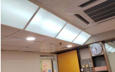
Facility Repairs in the Staff Canteen
