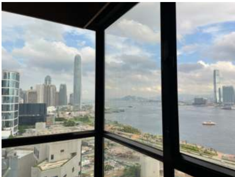
Double Glazing on the 14-21/F (20-21/F - Refurbished in 2016, 18-19/F - Refurbished in 2018)
