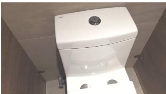
Dual Flushing Cistern
