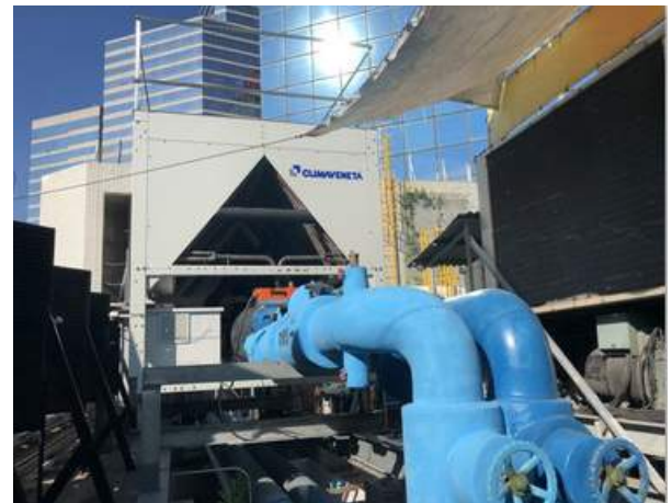
Oil-free Chiller, installed in 2018
