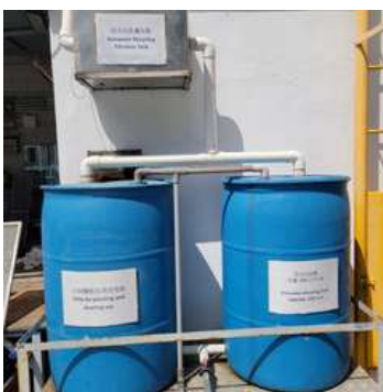
Rainwater Collection System
