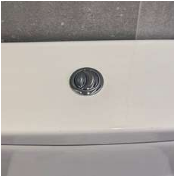
Dual Flushing Cisterns
