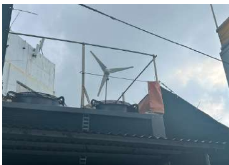
Install Wind Turbine on the Rooftop
